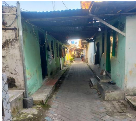
Figure 8. Condition of the access road to the Kampung Emas Bumijo settlement
